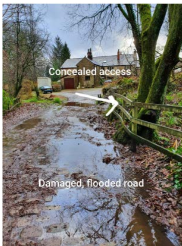
Image shows the concealed entrance to the proposed access road, access to Horrobin Fold, and the current damage and flooding
